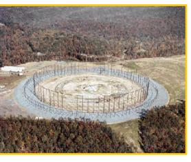
During the 1950s and 1960s, NRL demonstrated technology that permitted a radical improvement in the performance of high-frequency direction-finding (HFDF) networks and oversaw the deployment of this technology in Project Boresight and Project Bulls Eye.
