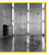
steel tanks. Each tank holds up to 300,000 barrels of aviation fuel, with the largest being 100 ft in diameter by 250 ft high. To give a better indication of the size of these fuel storage tanks, a 300,000-barrel tank holds enough gasoline to give a 12-gallon fill-up to 1,050,000 automobiles.
