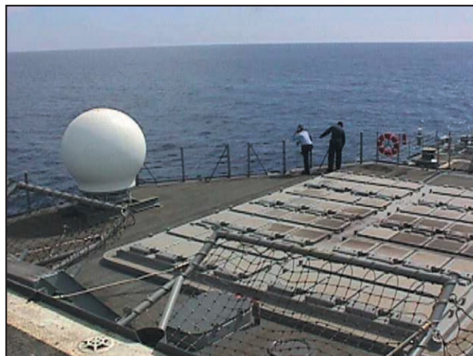
FIGURE 4 NRL installed high-data-rate SATCOM equipment like the antenna shown here on four Navy ships and two shore sites for FBE-India.
