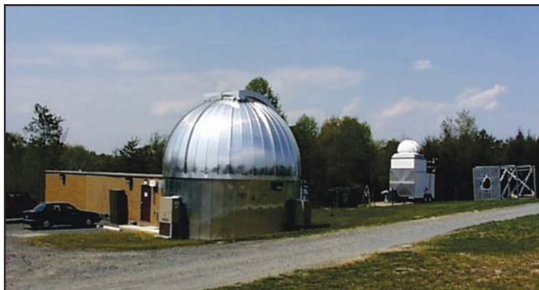
Naval Center for Space Technology Optical Test Facility at the Midway Research Center, Stafford County, Virginia. Large dome on the left houses a 1-m telescope with active laser transmit and receive capability. Smaller dome and trailer in background is a self-contained transportable 16-in. telescope that has been used as a passive optical tracker and a laser communications receiver.
