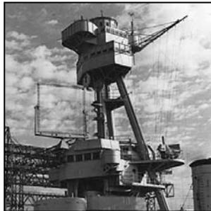
NRL invented and developed the first U.S. radar (1922–1939).
