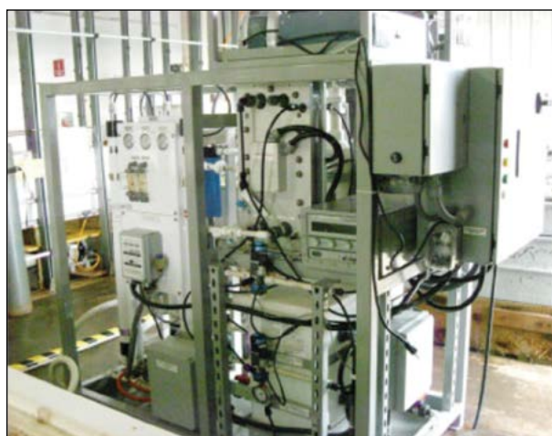
FIGURE 5 NRL electrochemical acidification carbon capture skid. The acidification cell is mounted onto a portable skid along with a reverse osmosis unit, power supply, pump, carbon dioxide recovery system, and hydrogen stripper to form a carbon capture system (dimensions 63 in. × 36 in. × 60 in.).
