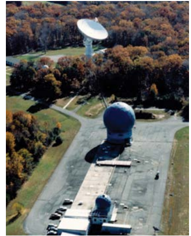
The NRL Pomonkey Facility.
