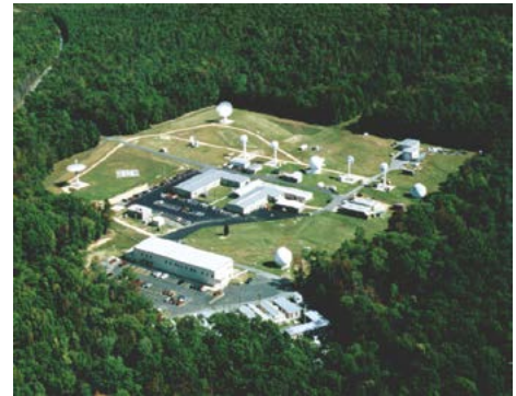
Blossom Point Satellite Tracking and Command Facility.
