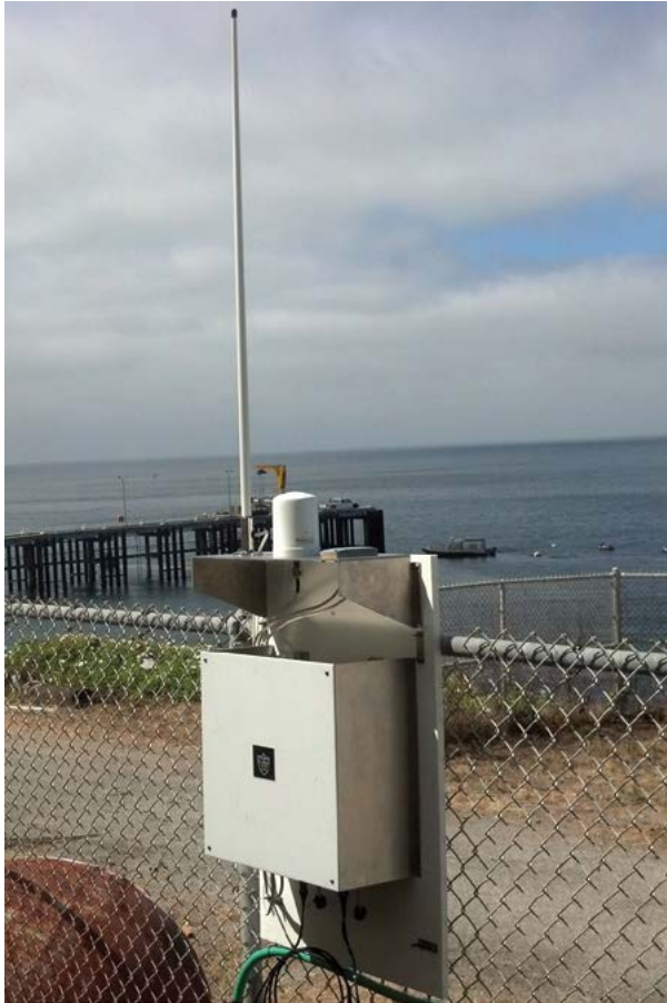
FIGURE 9 An installed RAIDER-M unit.
