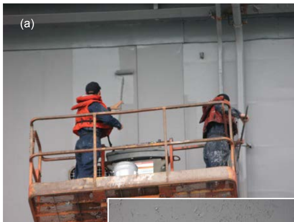
FIGURE 1 (a) Roll application of a silicone alkyd topside coating by Ship's Force, and (b) peeling/delamination of a silicone alkyd topside coating on a Navy ship.
