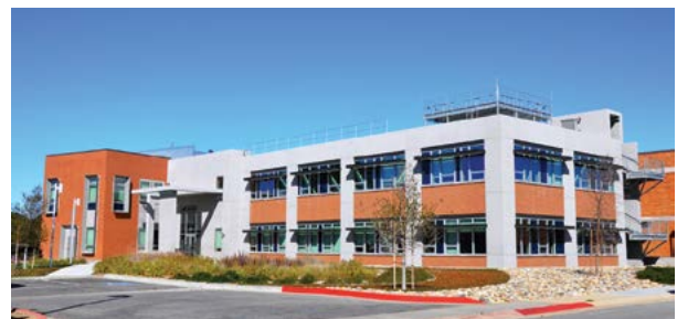
NRL Monterey's new 15,000 ft 2 Marine Meteorology Center. The building was constructed through the MILCON program, Project P-174, and was dedicated on October 12, 2012.
