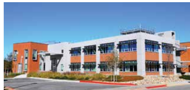
NRL Monterey's 15,000 ft 2 Marine Meteorology Center. The building was dedicated in October 2012.
