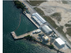
Marine Corrosion Facility Key West, FL
