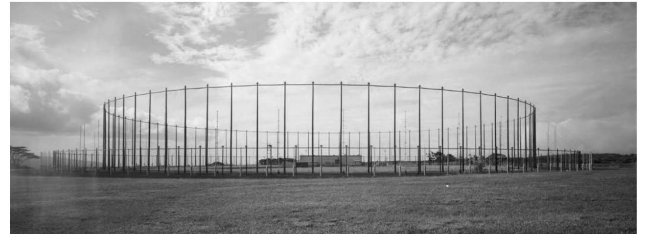
In the 1950s, NRL initiated "Project Boresight," a program that sought to make radical improvements in high-frequency, direction-finding networks. The AN/FRD-10 antenna, shown here at Naval Radio Station Pearl Harbor, was originally developed to pick up new advanced Soviet communications. Library of Congress photo
