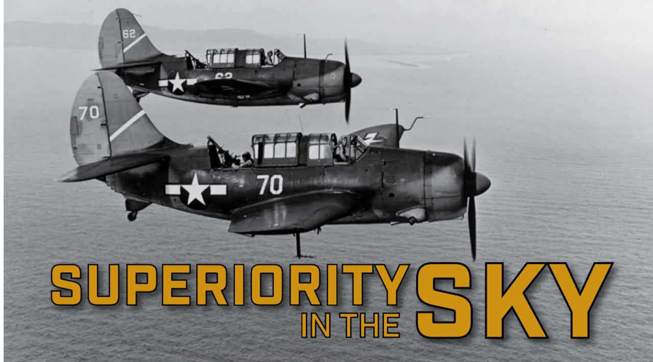
**NRL CONTRIBUTIONS TO AIR WARFARE INCLUDE THE DEVELOPMENT OF THE FIRST AMERICAN AIRBORNE RADAR, SUCH AS THIS ASB SYSTEM ON THE STARBOARD WING OF A WORLD WAR II HELLDIVER AIRCRAFT.**
