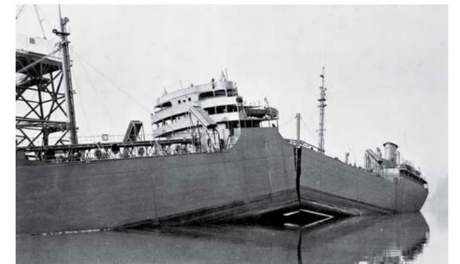
In the 1940s, NRL solved the mystery of brittle fractures of World War II Liberty ships, in which entire ships sometimes fractured, establishing techniques that are still relevant in the age of high-performance ships, aircraft, and missiles. NRL photo
