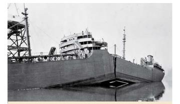
In the 1940s, NRL solved the mystery of brittle fractures of World War II Liberty ships, in which entire ships sometimes fractured, establishing techniques that are still relevant in the age of high-performance ships, aircraft, and missiles.NRL photo VOL. 9, NO. 2, 2023
