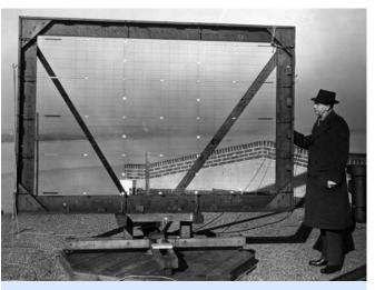
The first US radar tested for shipboard service, similar to this one shown in 1937, was installed aboard the destroyer USS *Leary* (DD 158) before a fully operational system was later put on the battleship USS *New York* (BB 34). NRL photo
