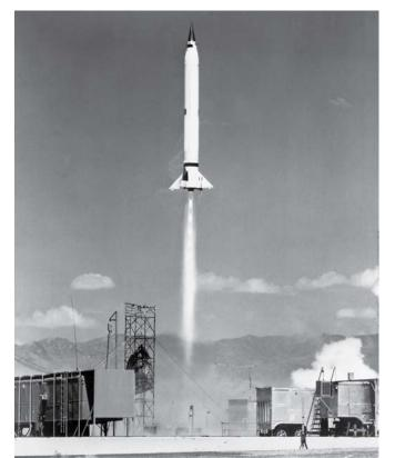
In 1946, NRL developed the Viking sounding rocket, the first rocket designed specifically for research purposes and the first to use attitude control. A total of 14 Viking rockets were launched by NRL between 1949-57. NRL photo
