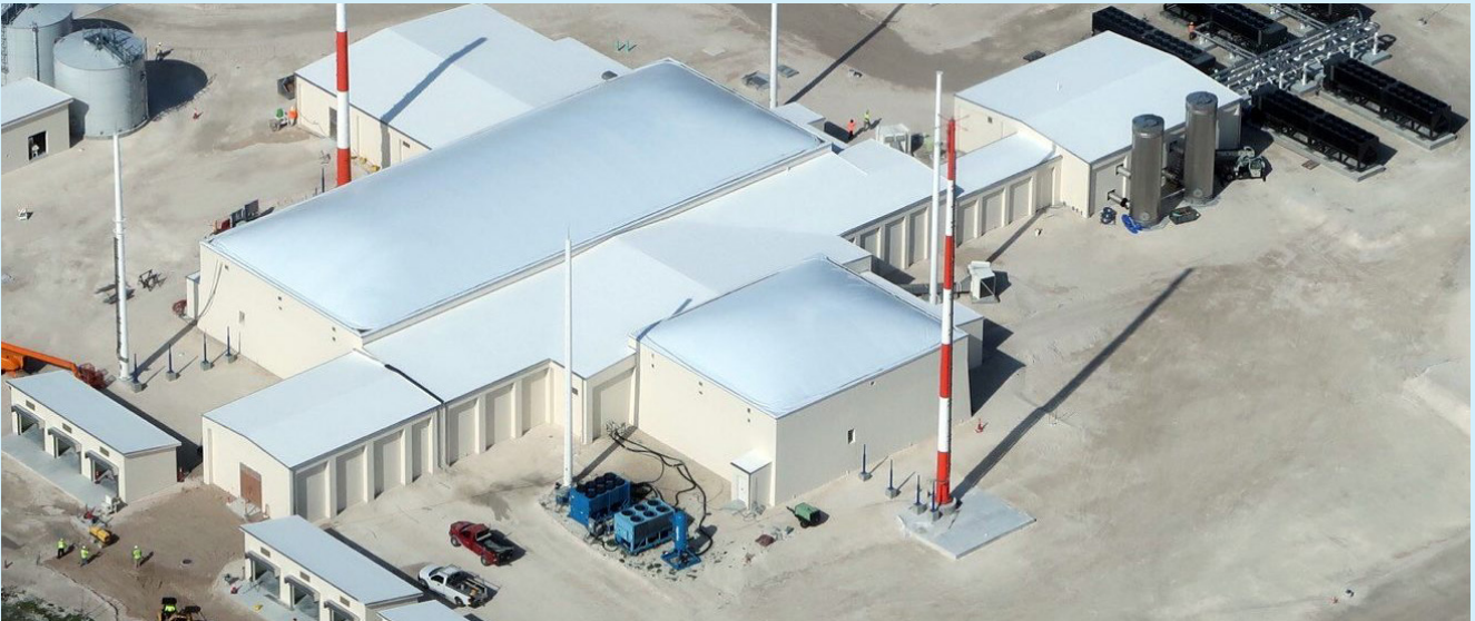
An aerial view of the Air Force's space fence under construction on Kwajalein Atoll in the Marshall Islands. Photo by Lockheed Martin
