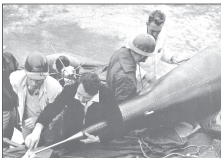
Angle-of-attack indicators are adjusted on the top of the nose cone. The silver Vanguard satellite is seen at left center. (NRL PAO-1963 (est.), Figure 2)
