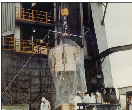
NTS-2 being lifted to the Atlas launch vehicle. (NRL Photo)
