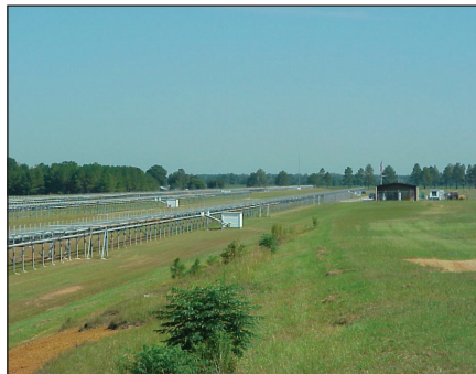
Antenna field at a Space Surveillance site. (NRL Photo)
