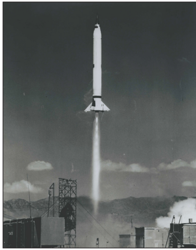
Takeoff of Viking 11, the heaviest Viking rocket ever fired, as it rose 158 miles to establish the altitude record for single-stage rockets. (Rosen-1955, p. 624)
