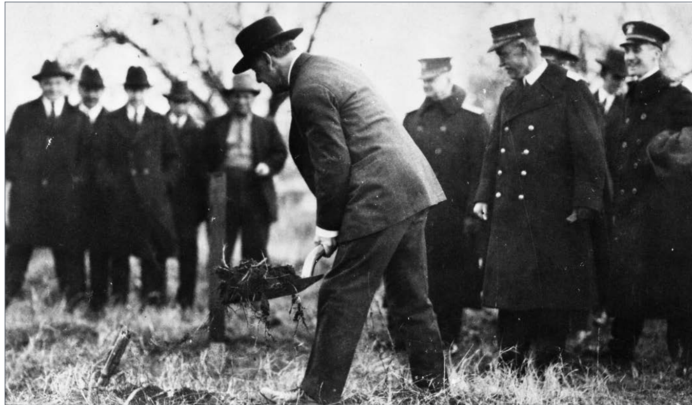
Secretary of the Navy Josephus Daniels breaks ground for NRL's first building on December 6, 1920.
