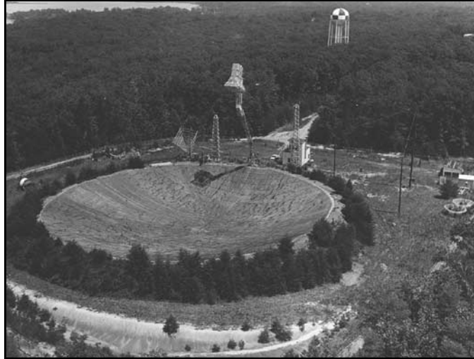
NRL built and used this 220-ft by 263-ft antenna in Stump Neck, Maryland, as part of a long-distance communication circuit involving Earth's natural satellite, the Moon, as the reflector of signals from the sender to receiver.
