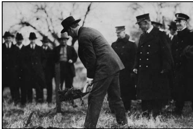
Secretary Daniels breaks ground for Building 1 in 1920.
