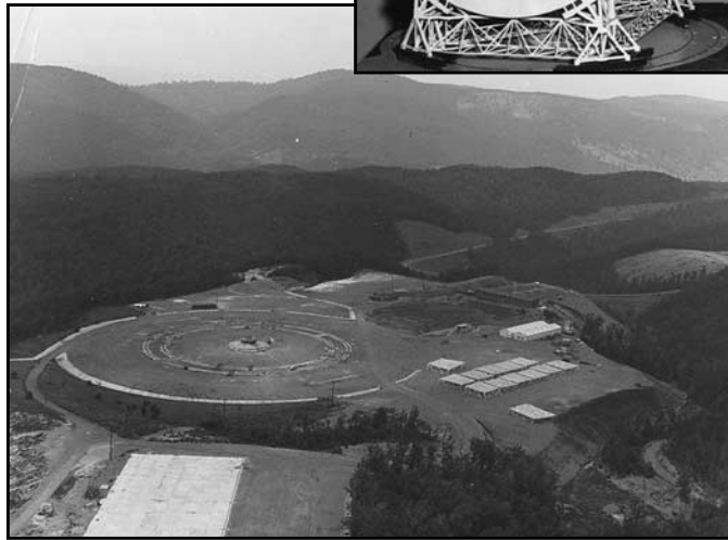
(b) Construction in Sugar Grove, West Virginia, began even before all of the engineering and design had been worked out.
